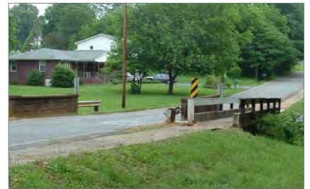
Above: Syphrit Road Pedestrian Bridge
