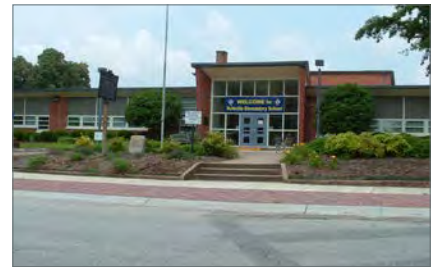
Above: Reidville Elementary
