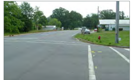
Above: Intersection of SC 9 and Hillbrook Circle/Church St.
